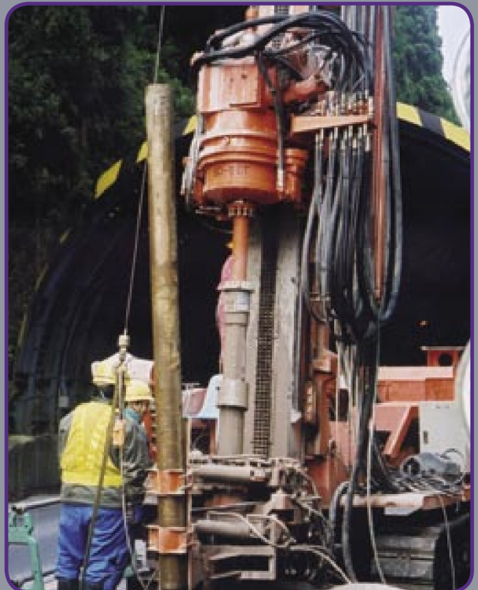
■ Drilling for the installation of geo-exchange tubing at a highway tunnel entrance.
