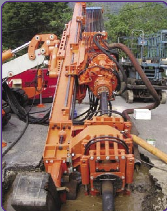
■ Installing tie-back anchors for a retaining wall.
