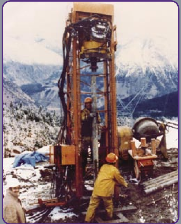
■ Installing combination micro pile and tension anchors for hydro-electric transmission towers in unstable ground conditions.
