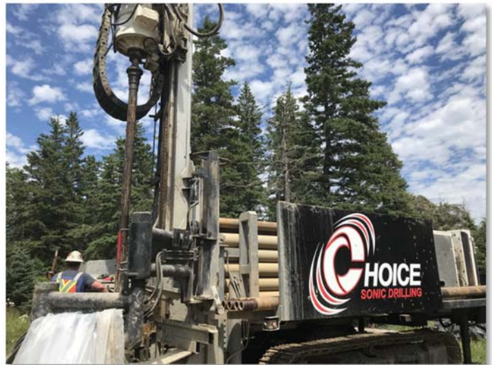
Drilling onsite with Choice Sonic Drilling.
